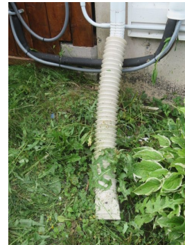
Downspout extension at back left corner
