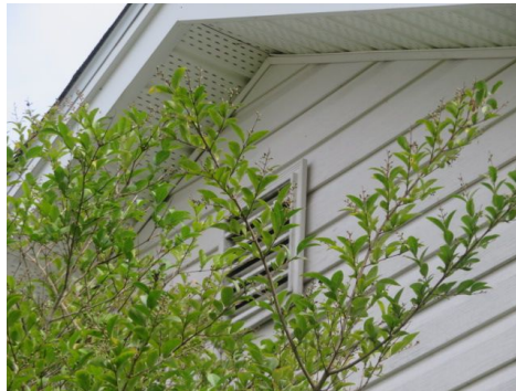
Right gable vent
