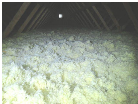
Loose fill fiberglass insulation
