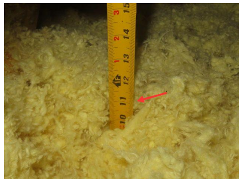
Insulation depth (avg. 11")
