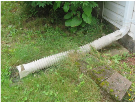
Extension at front left corner
