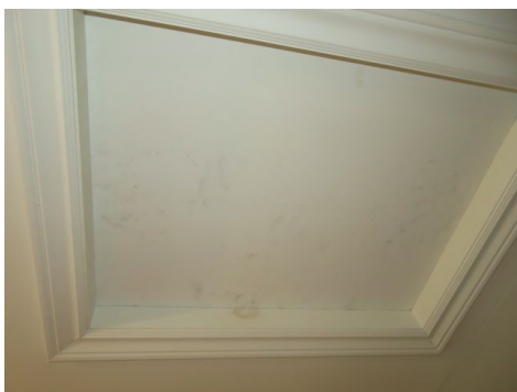
Attic access from Bedroom 2
