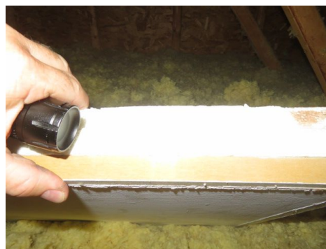
Attic hatch cover
