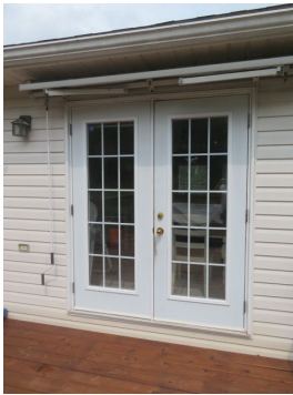
Patio doors to deck
