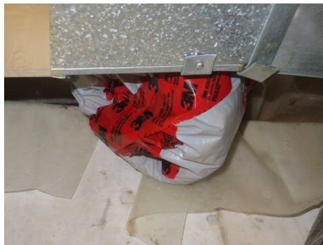
Combustion air supply not required
