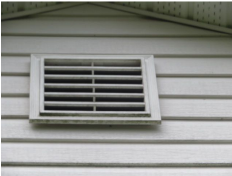
Left gable vent
