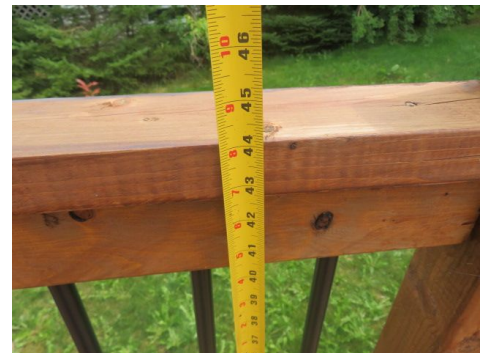
Deck railing height acceptable
