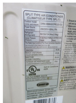
Heat pump outdoor unit nameplate
