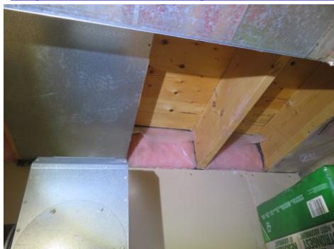
Insulated rim joist
