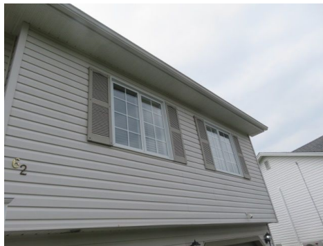
Front right windows
